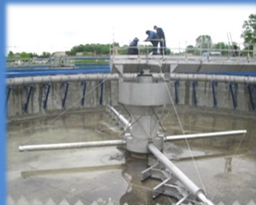
ASPIRATED SCRAPER BRIDGE WITH SIPHON - PARS
